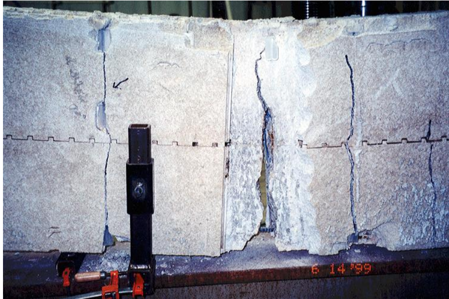
Figure 5c Typical Failure Mode for the Long-Span ICF Flat Lintel (4x24 specimen with foam removed at primary failure location)
