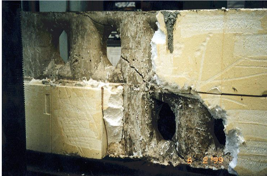
Figure 7b Typical Failure Mode for the Long-Span ICF Screen-Grid Lintel (6x24 specimen with foam removed from primary failure location)
