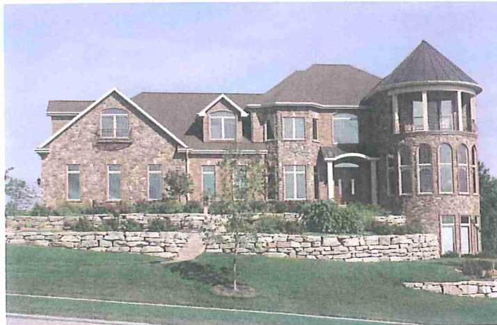
TF System utilized its vertical IFCs for this residence in Appleton, WI.
